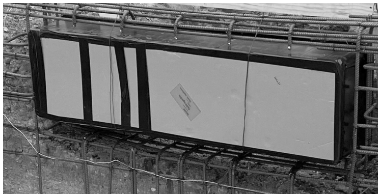
Image 4 BaduJet Turbo - Jet placement in rebar
