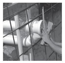
Figure 5 BaduStream *Single* Housing Installation
