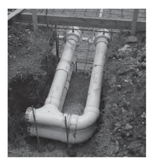
Figure 6 BaduStream **Dual** Housing Installation
