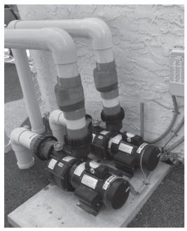
Figure 8 Check Valves Installed
