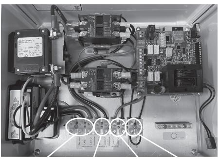
Power from main panel (230 VAC): Neutral, Line 1, Line 2 Power to pump motor 1 (230 VAC): Load 1, Load 2
